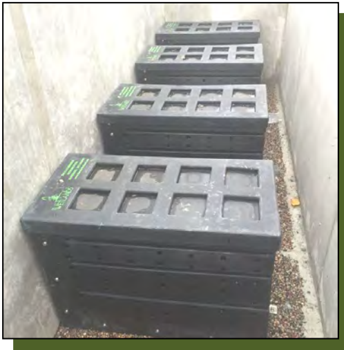
Pre-filter cartridges with tops on.
