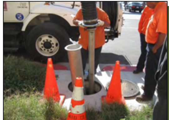
Insertion of vacuum hose into separation chamber.
