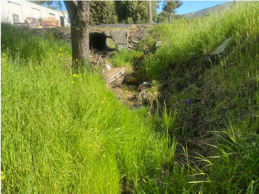
Photo 10. View from within the channel looking upstream at the culvert, with concrete slope protection around it. The tree is the same red willow as in Photo 9.
