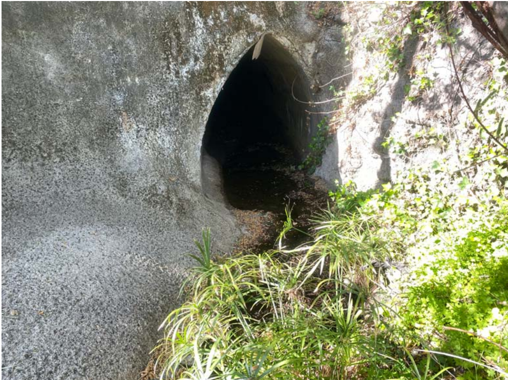
Photo 14. View of the culvert on the downstream side of the drainage with concrete slope protection. From this point the drainage runs under an industrial complex offsite.
