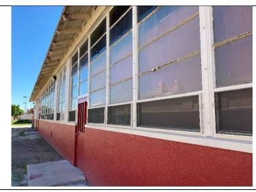
Photo No.6 – View of weathered window caulking.
