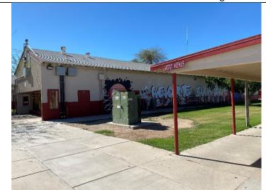
Photo No.7 – Pad-mounted electrical transformer located between High School buildings.
