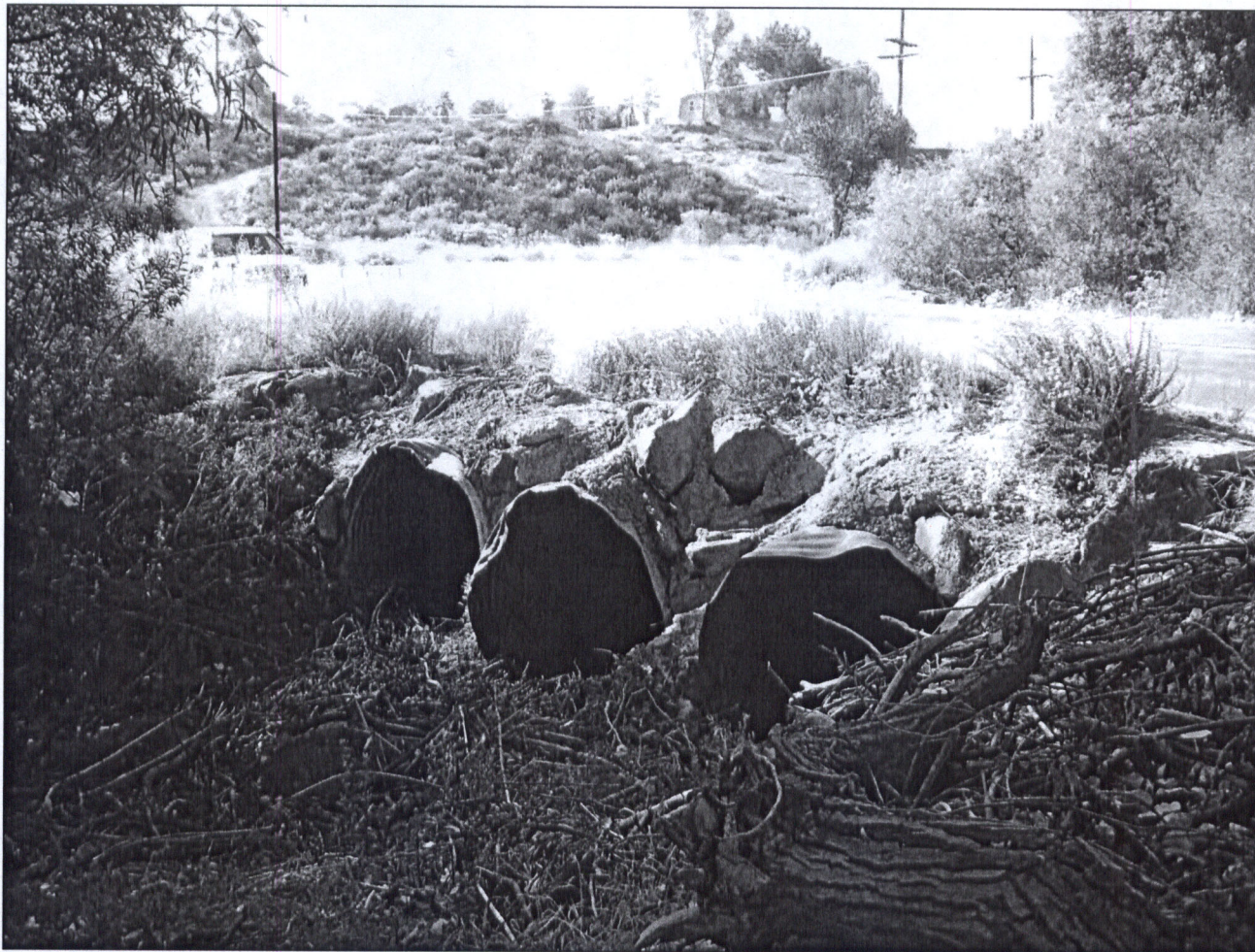
Figure 3. Modern, large-diameter corrugated metal pipe culvert under a segment of Los Alamos Road where it crosses Warm Springs Creek (view to the south; photograph taken June 24, 2014). These culverts were added in 1987 when the road was paved.
