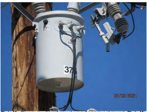
**Photo 16** - Closeup view of transformer shown in the previous photograph (**Photo 15**). No evidence of leakage was observed.
