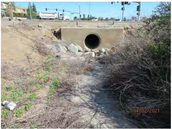
**Photo 6** - View to the north showing the concrete pipe, headwall, and concrete-lined channel in the northwest corner of the subject site. Minor windblown trash is visible.
