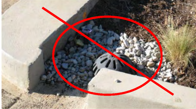
Figure 6: Incorrect Placement of an Overflow Inlet
