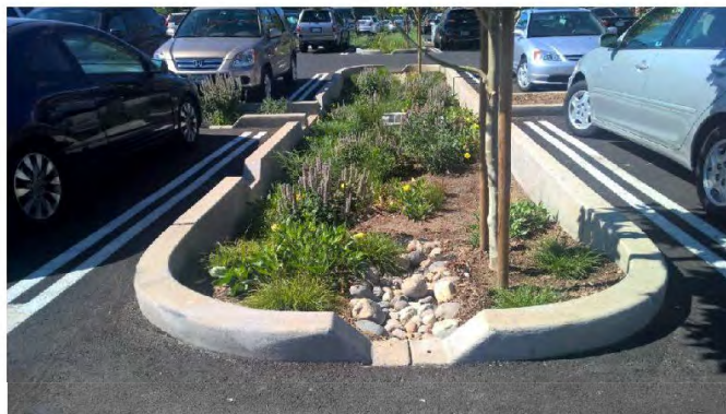
Figure 3: Curb Cut located in a Bioretention Facility
