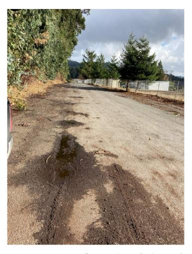
Image 8. Representative of RS2 conditions (looking east) near intersection of Chambers Road and Mattole Road. Details asphalt surface, 25'+ average road width, shoulders, turnouts, crowned geometry with fair drainage, average slopes <5%.
