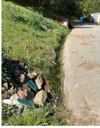
Photo 7: View of landslide repair at the base of 738 Loma Court. Water is actively seeping out of the sub drain outlet.
