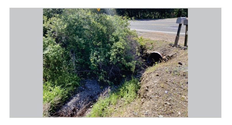
Inlet of existing 36-inch CMP (south end of roadside ditch), looking southeast (April 2022)
