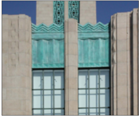
Pilasters extend past parapet
