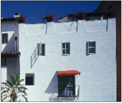
Roof as balcony behind articulated parapet
