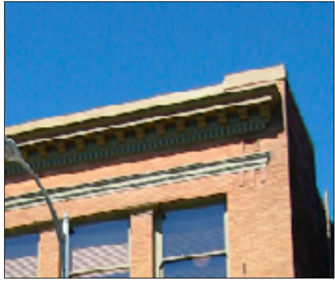
Cornice of cast concrete with brackets
