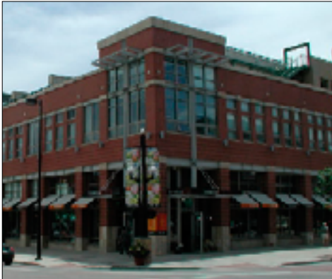
Flat roof with precast concrete parapet
