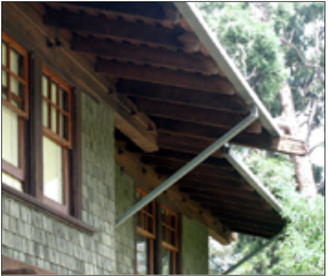
Large overhanging eaves with exposed rafters
