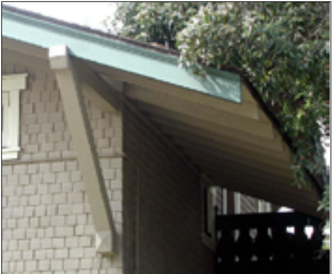
Brace and exposed rafters
