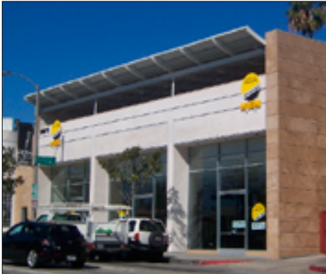
Curved metal roof covering outdoor roof deck
