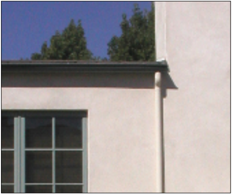
Gutter and downspout
