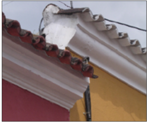
Terra cotta tiles on profiled parapet
