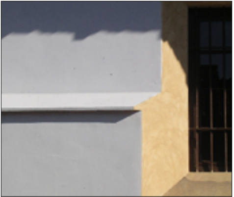
Intermediate molding at base
