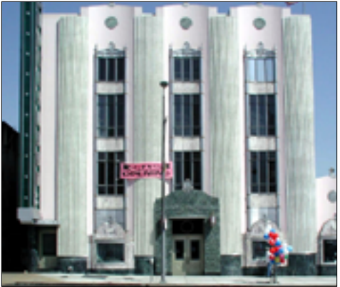
Plaster walls and pilasters with metal windows
