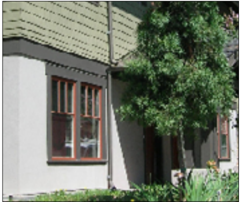
Stucco base with stained wood shingle wall
