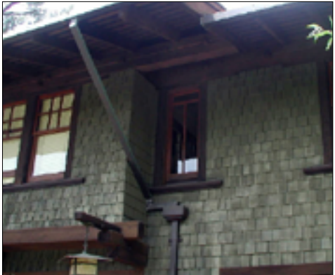
Gutter and downspout
