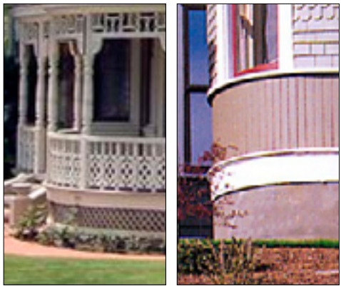
Base - wood trim & lattice, wood siding over stucco
