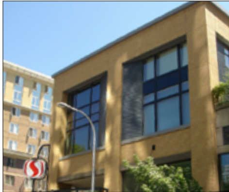
Simple brick pattern beneath parapet cap
