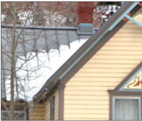
Metal Roof - standing seam, cross gable roof
