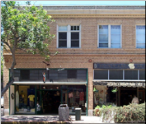
Wall with base, middle, top articulated in brick
