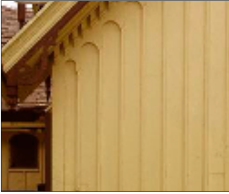
Board & batten wood siding
