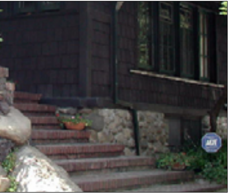
Tapered stone foundation base, shingle wall
