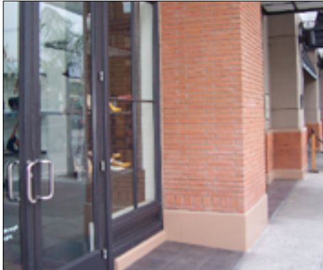
Concrete base with brick columns and walls
