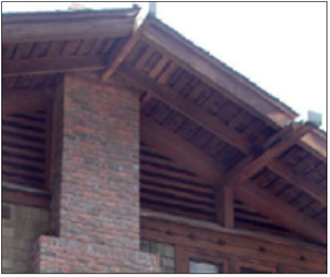
Structural elements expressed at gable end vents
