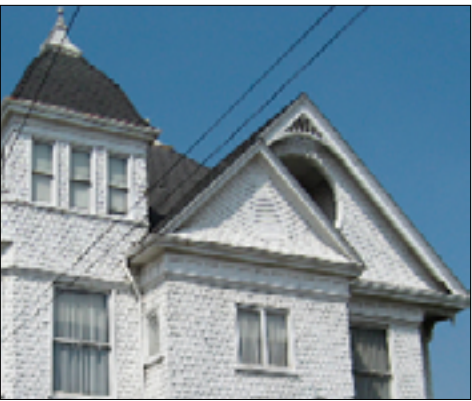
Closed gable ends with shingle patterns
