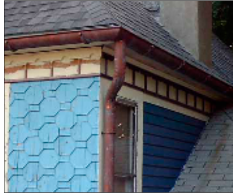
Gutter - half-round w/ brackets, downspout
