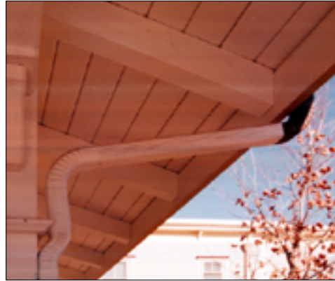
Gutter and downspout
