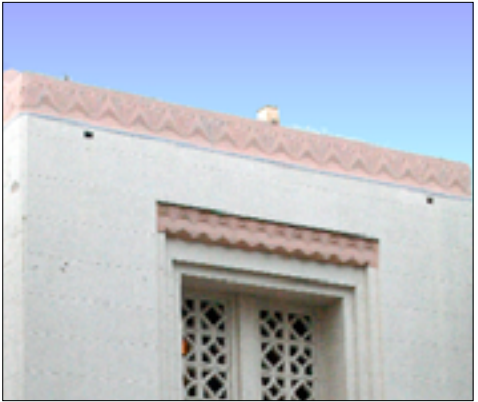
Roof overflow scuppers recessed into facade
