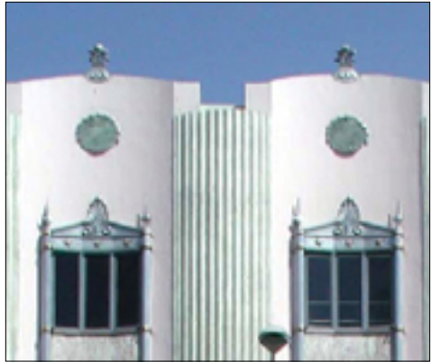
Stepped parapet w/ crenellated pilasters
