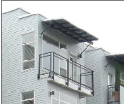
Metal Awning with exposed rafters
