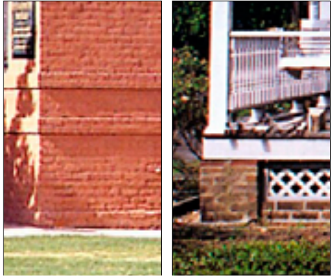
Base - brick, brick pier & lattice infill
