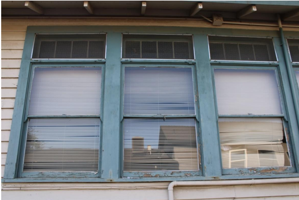
Figure 11. Unaltered windows on the east elevation, with horn stiles on double-hung windows.
