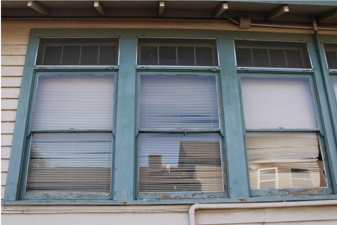
Figure 29. Unaltered windows on the east elevation, with horn stiles on double-hung windows.
