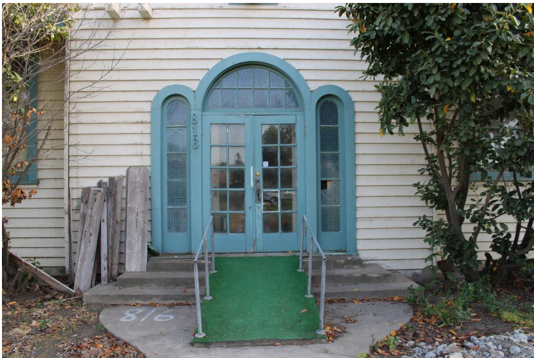
Figure 21. Arched front entry with double divided light doors, and side lights, facing south.
