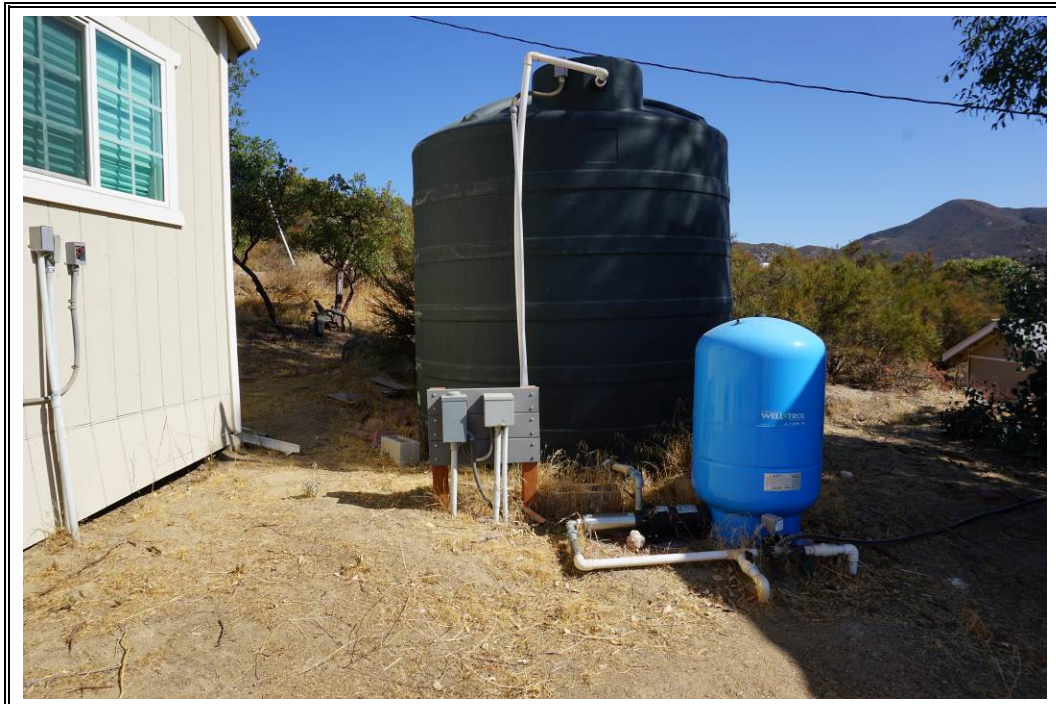
Photograph Number 9: View of aboveground storage tank (AST) and expansion tank associated with the groundwater well located on the northern portion of the subject property, facing north.
