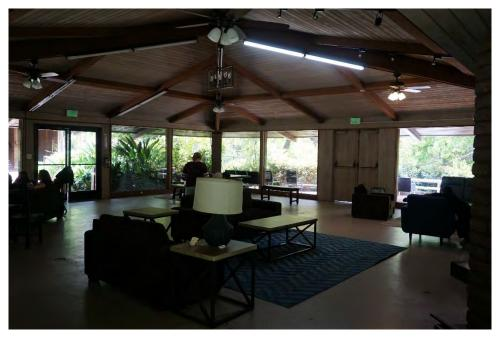
Photograph 22. Interior photograph from 2018 showing exposed wood beam ceiling and continuous window walls
