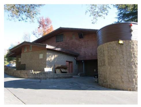
Photograph 30. Overview of rear (west) elevation showing extensive use of split-face CMU, view to east
