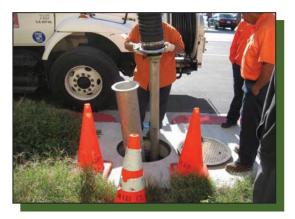
Insertion of vacuum hose into separation chamber.
