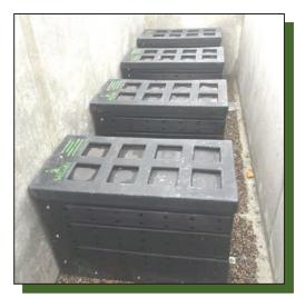
Pre-filter cartridges with tops on.
