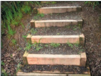
Example of a cribbed staircase
