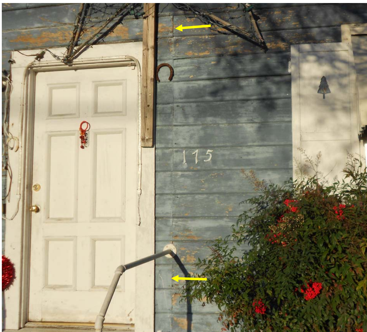
Photograph 175 Monroe Street View: Front door showing the scars from the original opening and the remodeled door system. Window shutters, pip railing and concrete steps, are also not original.
