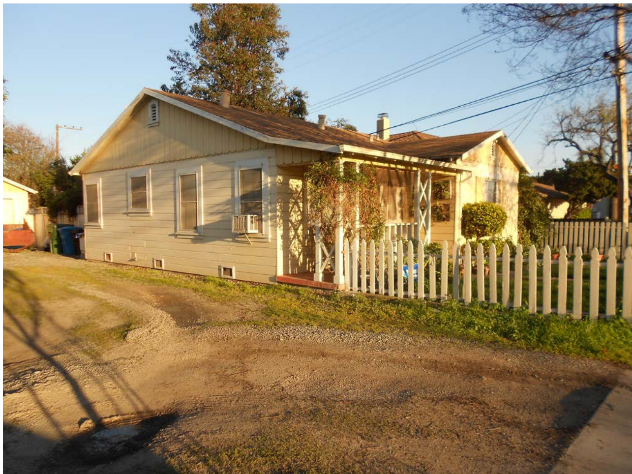
Photograph 2 171 Monroe Street View: west façade of the house showing the intersecting gable roof, the fenestration and the porch.
