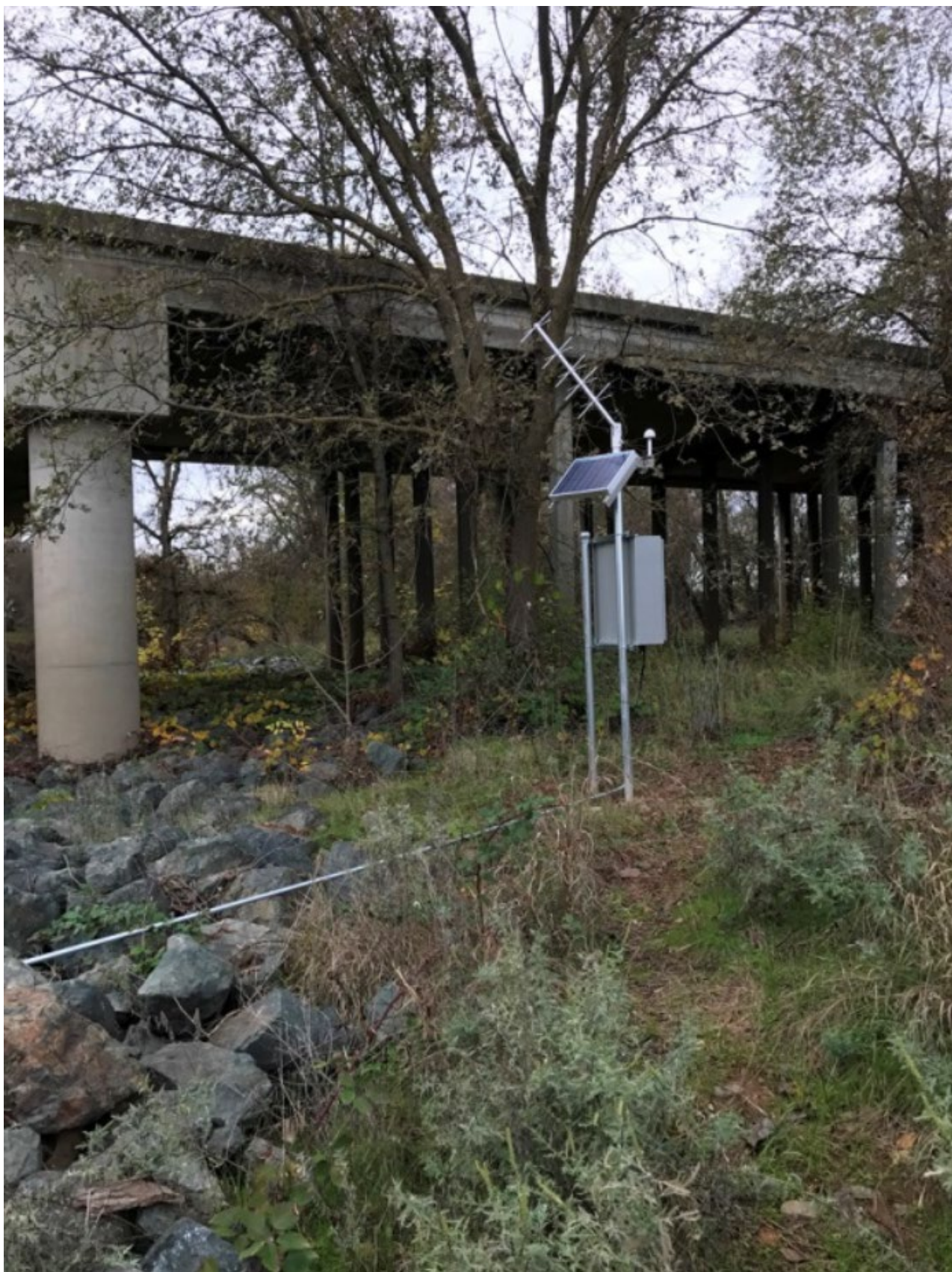
Figure 7. Example of a typical constructed RTU enclosure with an antenna/solar panel mast.
