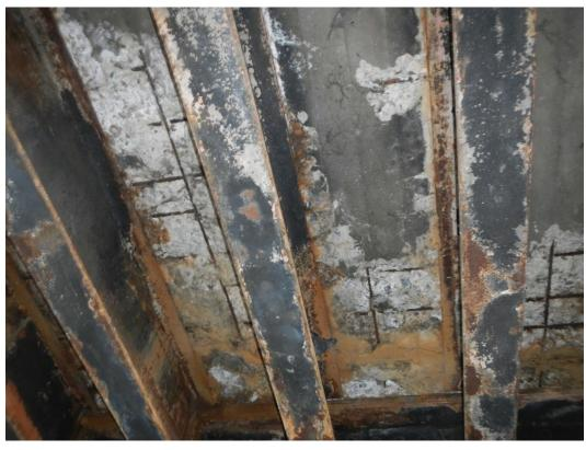
Figure 3. Spalling Concrete Deck and Corroded Steel Reinforcement
