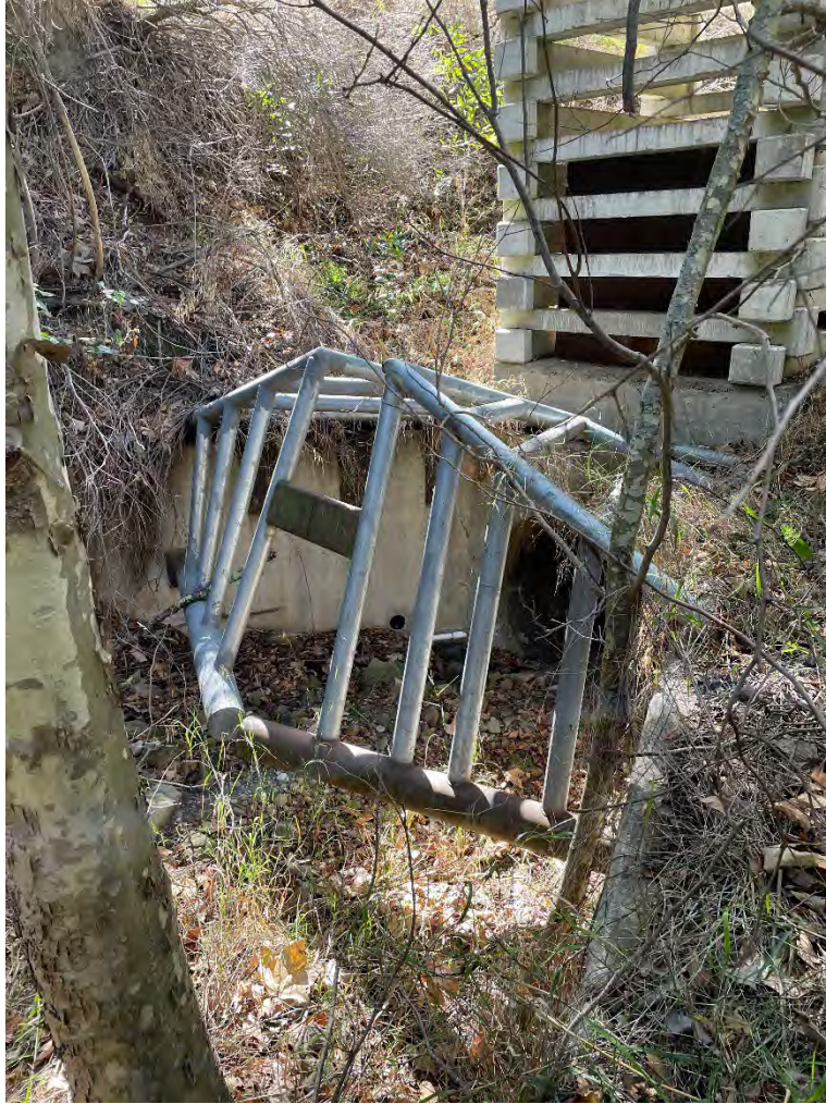
Photo 13. At PM 25.70, the culvert inlet has a trash rack and a debris box stand structure. Vegetation nearby includes sycamore, bay, and oak. October 27, 2021.
