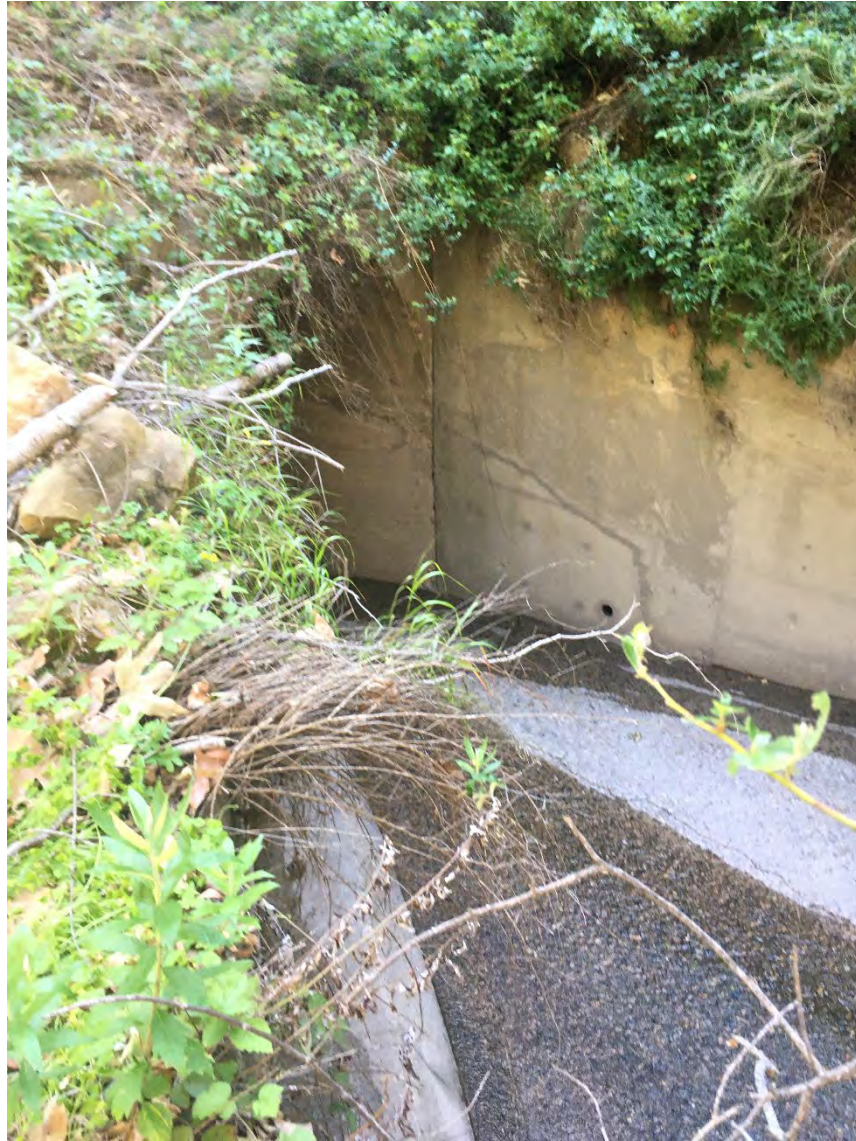
Photo 19. PM 27.67 culvert inlet with concrete apron and wingwalls. April 15, 2021.
