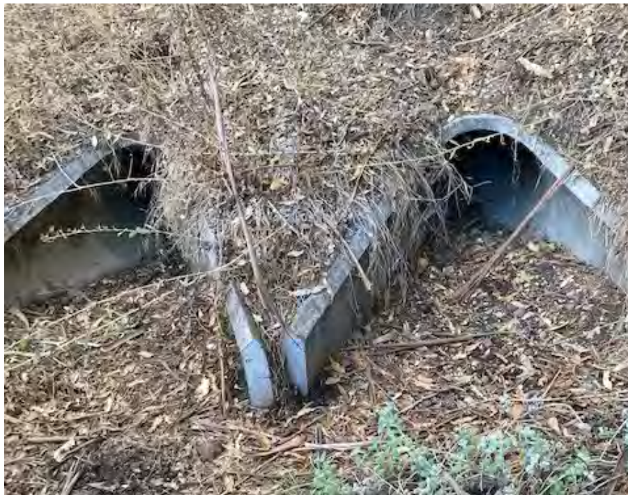
Photo 2. Inlet of culvert at PM 6.87. Note debris and sediment buildup. March 24, 2020.
