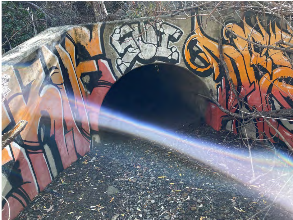
Photo 8. The PM 22.0 culvert outlet has a headwall and wingwalls. The pipe is partly filled with sediment. October 27, 2021.
