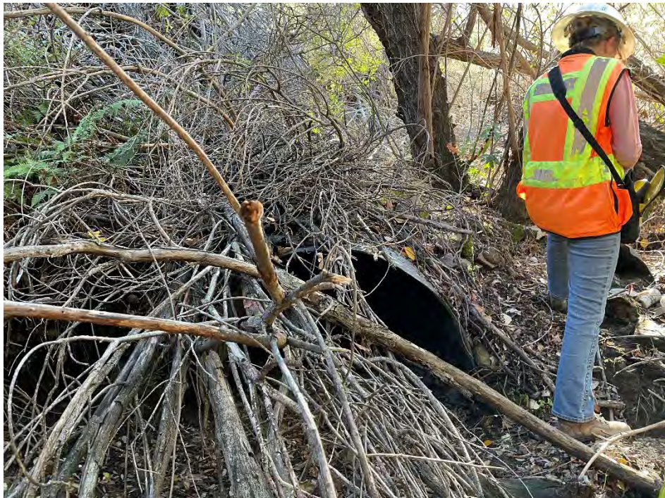
Photo 6. The culvert at PM 21.57 outlets into a channel with a mud bottom. Some dead brush and debris partially obscure the outlet. Red willow and arroyo willow are present on the banks. October 27, 2021.
