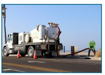
The average maintenance time is 45 minutes using a standard vacuum truck.
