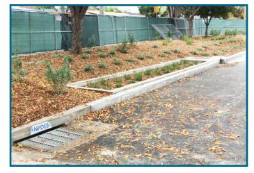
All-in-one treatment train, no need for separate trash capture manhole or vault.
