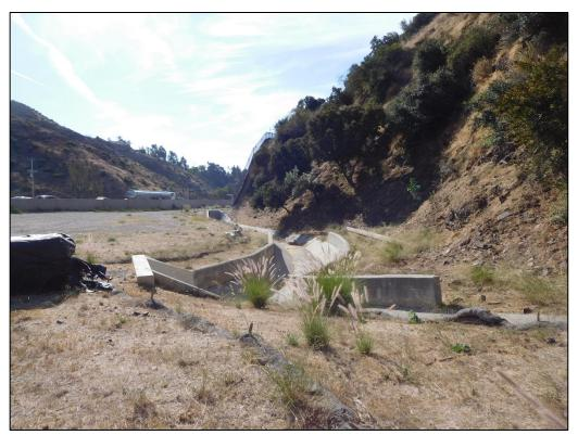
Photo 7. Trapezoid Channel and Headwall North of Caltrans Retaining Wall Adjacent to Oak Parking Lot B, View Facing Southeast
