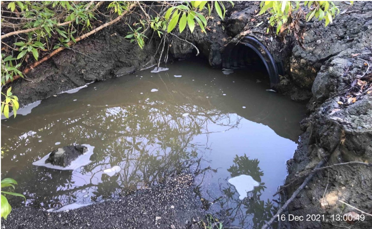
Photograph 10. View of the culvert that conveys water from beneath Pillar Point Harbor Boulevard to Pillar Point Harbor. The drainage is surrounded by several arroyo willows.
