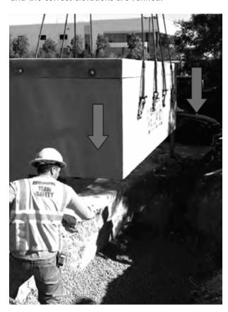
Once the vault is set in place, check all four corners are in the correct position. Take tension off of the rigging to ensure the vault is set properly and the compacted rock backfill below is holding the weight of the vault.
