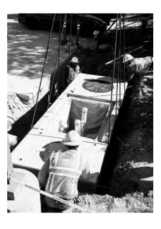
7. Use a string and or level to make sure the vault is level in both directions. The vault cannot be more than 0.5% slope off from level in any direction. If the vault slopes more than 0.5%, pick back up, move to a safe area, re-level the rock below and reset until properly level.
