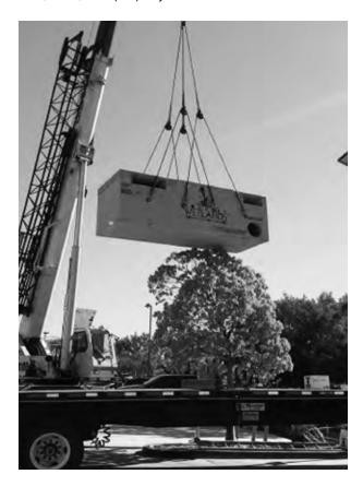
5. Position the concrete vault over the excavated area and slowly lower into position. Ensure the inlet and outlet sides of the vault are in the correct position and the correct elevations are verified.
