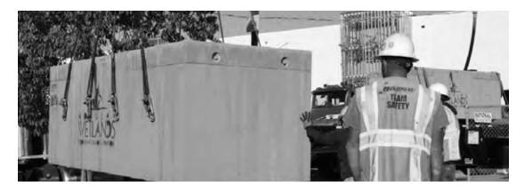
The contractor is responsible to provide the appropriate rigging and lifting connectors. Spreader bars are recommended to prevent damage to the concrete vault. All lifting points on the concrete vault must be used for safe offloading. Guide ropes can be used to stabilize the vault during offloading.
