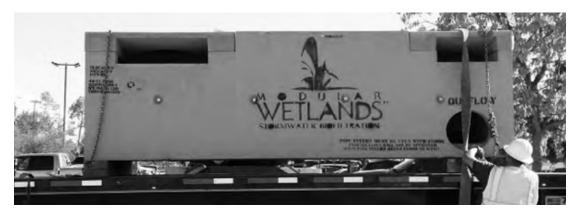
Position crane in a safe and optimal position for unloading. Ensure that the crane operator has the proper weights and distance to install location to allow for proper setup. The crane operator will provide instructions to the delivery driver on where to position the truck for offload.
