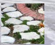
Permeable pavement allows water runoff to infiltrate through the soil and prevents most pollutants from eaching the storm drain system.
