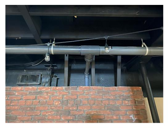
Photograph 20. Example of SSDS piping (06/01/2021).
