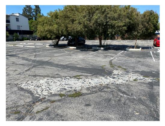
Photograph 33. Asphalt pavement in the southern portion of the Site, in poor condition (06/01/2021).
