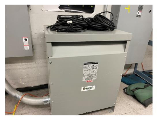
Photograph 14. Small dry-type electrical transformer located in the equipment room (06/01/2021).
