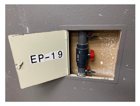
Photograph 15. Example of an Extraction Point (EP) for the sub-slab depressurization system (SSDS) (06/01/2021).
