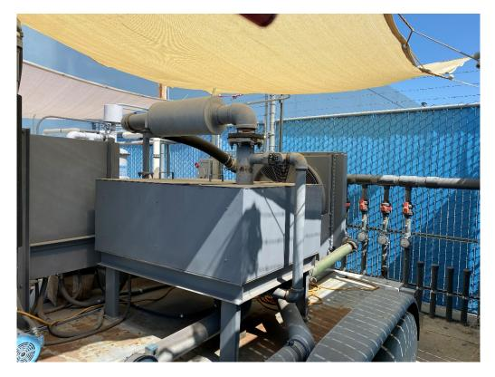
Photograph 41. Equipment inside the enclosure for the SSDS and Soil Vapor Extraction (SVE) system (06/01/2021).
