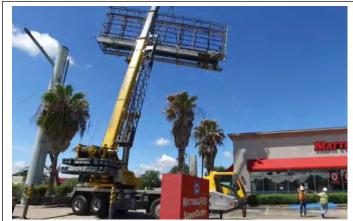
The proposed Project would involve the demolition of the existing pole sign structure and would include the use of a hydraulic truck crane and other heavy equipment during the construction and installation of the proposed digital sign.
