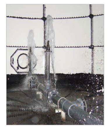
In circular, rectangular and irregularly-shaped reservoirs, the diameter or length is greater than the depth. A single fixed-diameter inlet pipe (common or separate from outlet pipe) results in short-circuiting, poor mixing and dead zones in areas away from the inlet because the momentum is concentrated in one localized area of the tank.
