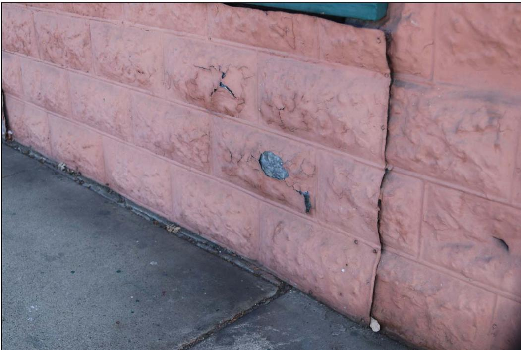
*Photo 36: West elevation, condition of pressed tin*
