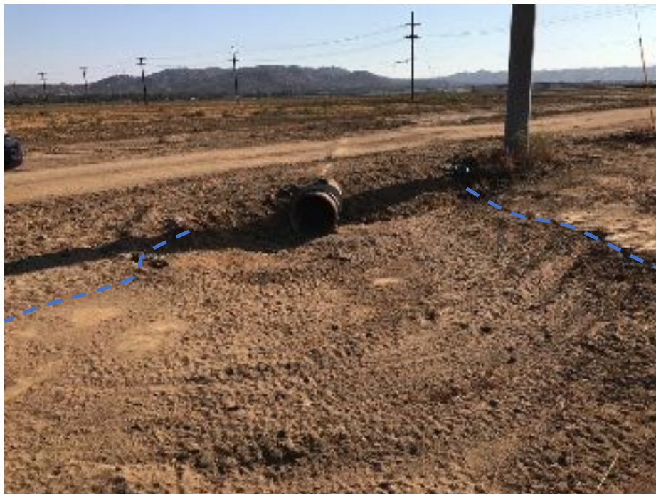
Photo 12. Upstream view of a culvert road crossing within Feature 2. The project site contains two centrally located parallel roads that run from the western to eastern project boundary. Feature 2 drains from this culvert outlet onto the southernmost road and continues west along the road into a set of storm drains on the western project boundary. Photo taken facing northeast.
