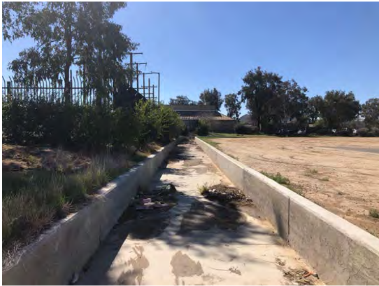
Photo 25. View of ODP 6, facing south, within Ditch 5. ODP 6 contained debris present as sediment and dead plant material one day after a rain event; however, Ditch 5 did not exhibit any other OHWM indicators (33.742870, -117.152704). February 24, 2022.
