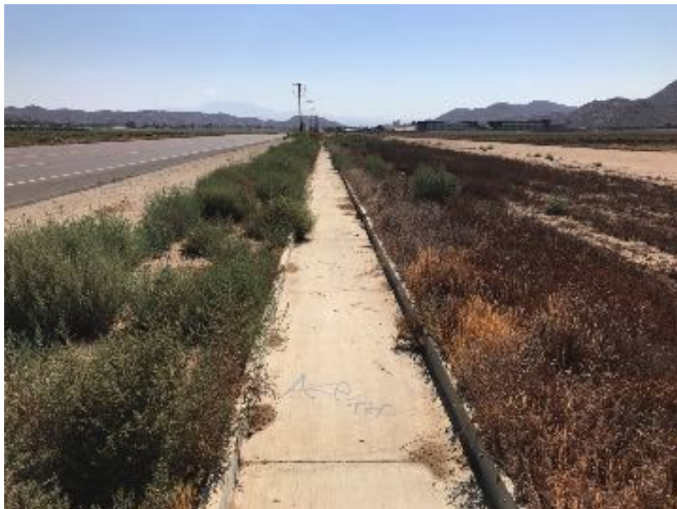
Photo 14. Upstream view of Ditch 1, along CA-74. The feature is concrete-lined for approximately 1,263 linear feet. Photo taken facing east.
