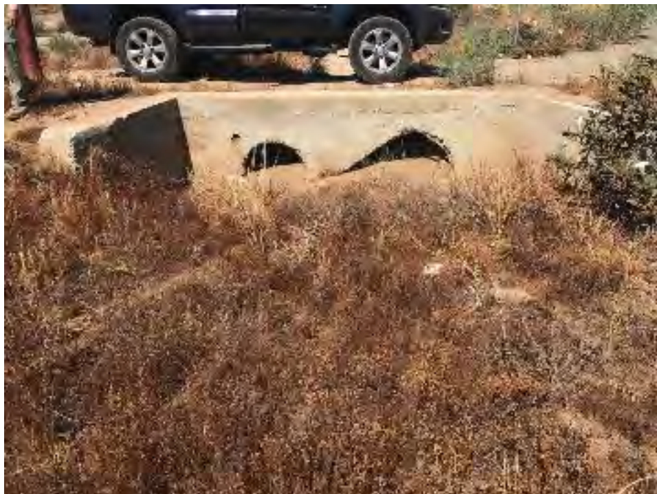
Photo 16. Downstream view of Ditch 1, along CA-74. The feature flows to this culvert for approximately 509 feet and is concrete-lined on the other side. Photo taken facing west.
