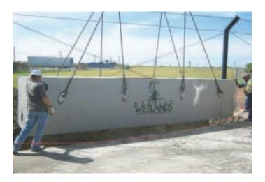
The MWS Linear is simple, easy to install, and has a space-efficient design that offers lower excavation and installation costs compared to traditional tree-box type systems. The structure of the system resembles precast catch basin or utility vaults and is installed in a similar fashion.
