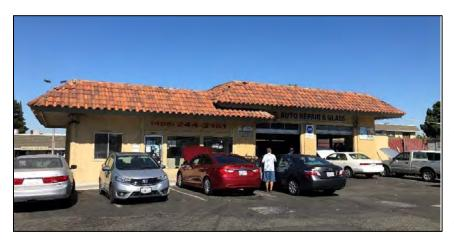
The canopy, which also has a mansard roof with clay tile, shelters the location of the former gas pumps.
