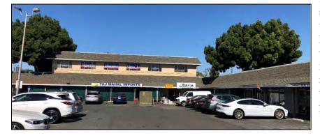
and has wooden board and batten cladding on the walls on the ground floor below the storefront windows. A mansard-like<sup>19</sup> asphalt shingle-clad structure functions as a parapet and hides the flat roof that covers most of the structure at the first floor. An asphalt shingle-clad mansard roof tops the second floor and hides the mechanical units on the roof. The east and north façades of the complex face narrow vehicle access ways which are also used for parking.
