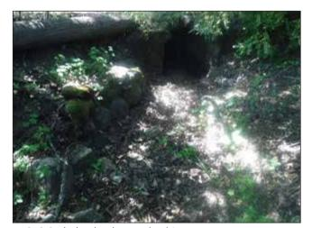
PHOTO 6: 3'x3' arch culvert under driveway
