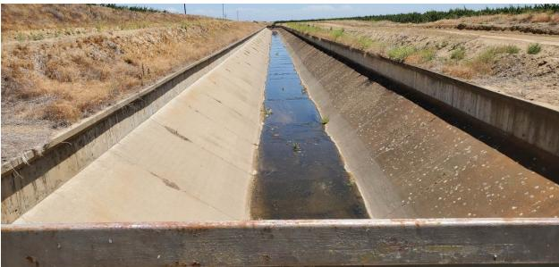
Photo 8: The concrete lined Newman Wasteway within the project APE.
