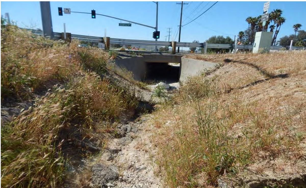
**Photograph 4.** View south and downstream of the roadside drainage channel showing the single box culvert under Spruce Avenue near the Redlands Boulevard and Spruce Avenue intersection.
