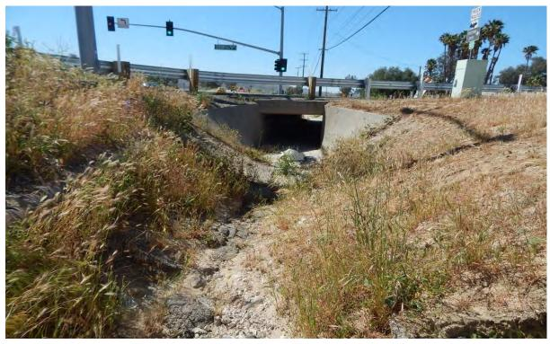
**Photograph 4**. View south and downstream of the roadside drainage channel showing the single box culvert under Spruce Avenue near the Redlands Boulevard and Spruce Avenue intersection.
