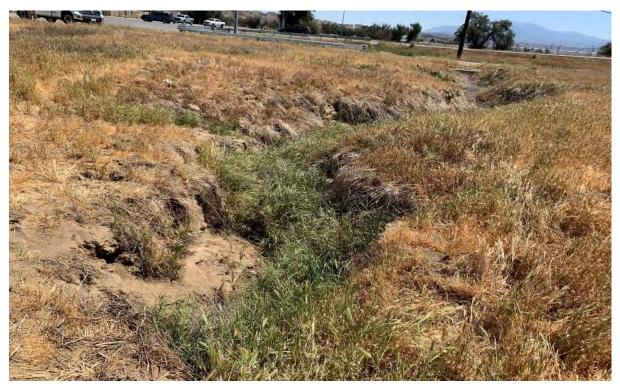
**Photograph 6**. East-facing view toward Spruce Avenue and Redlands Boulevard intersection showing weak water flow evidence and dense annual grasses in the erosional drainage ditch.
