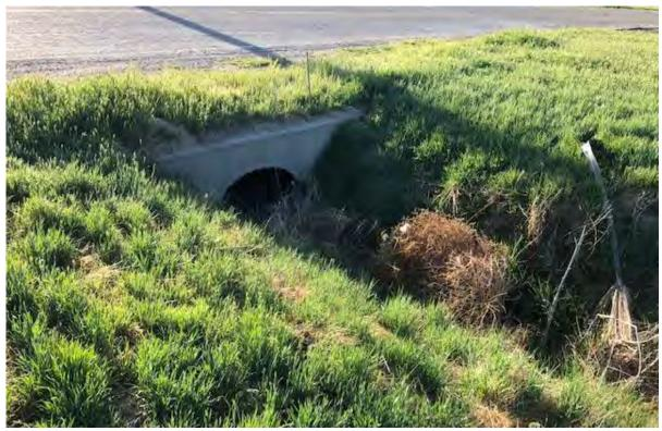
**Photograph 7.** Showing where the erosional drainage feature meets the culvert under Spruce Avenue.
