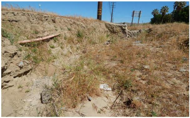
**Photograph 3**. View north and upstream of the roadside drainage channel showing the low-flow channel to the left of a terrace, steep banks, and a drop weir structure in the channel bed in the background.
