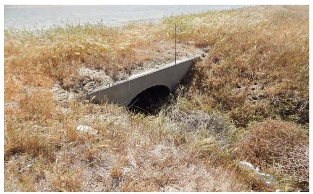
**Photograph 8**. Showing single storm drain intake under Spruce Avenue and Russian thistle in the channel bed at the downstream east end of the erosional drainage ditch.
