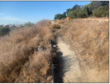
Photo 8: Close-up view of the concrete drainage ditch connection within the project site.
