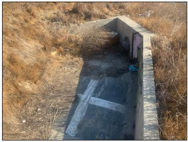
Photo 7: Close-up view of the concrete drainage ditch connection to the corrugated metal pipe storm drain.
