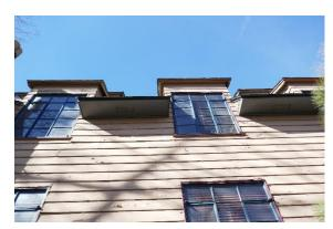
Figure 15: Detail of windows and boxed eaves at plan east façade.
