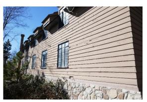
Figure 16: North end of plan east façade with peeling paint, looking southwest.
