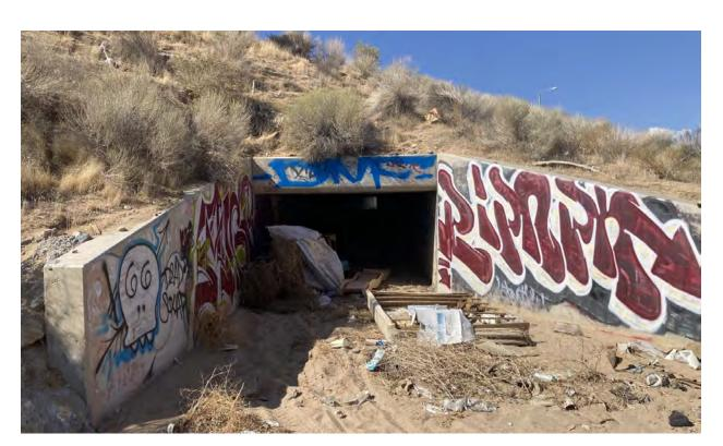
Photograph 4: Photo looking southwest within Drainage B near southern perimeter of the Project site. Photo depicts box culvert that conveys Drainage B beneath Ottawa Street.
