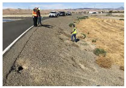
At Clifton Court Forebay Dam: Rodent burrows, slumping, and erosion due to animal burrowing, November 2019.
