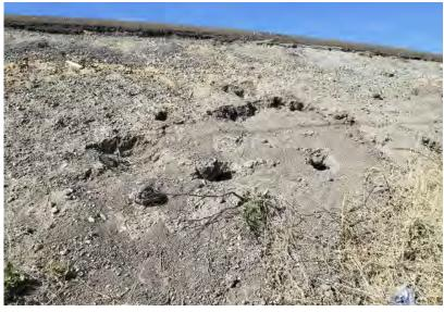
At Patterson Dam: Burrow holes and associated embankment surface slope failures on downstream dam embankment, November 2019.
