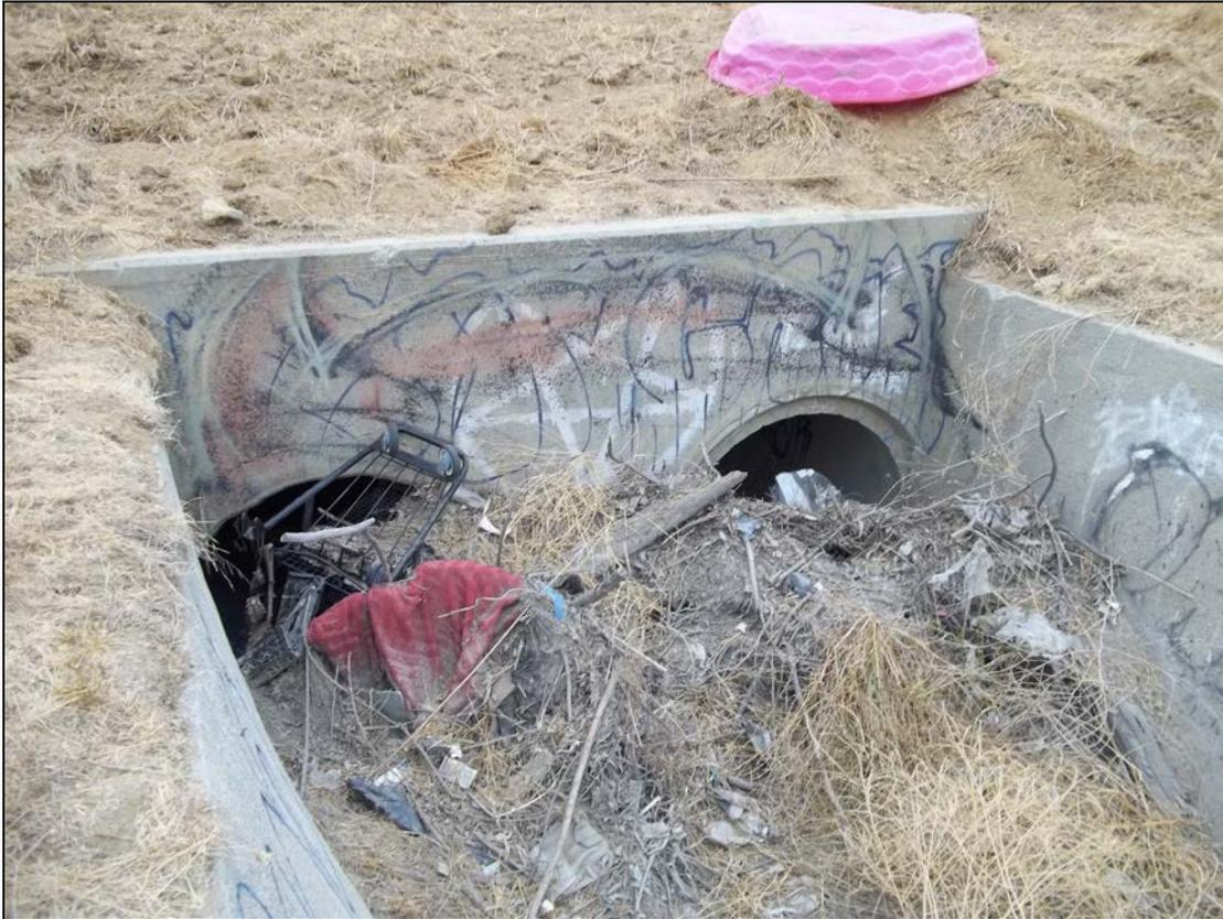
5. Northwest end of exposed ditch, two concrete culvert openings are visible
