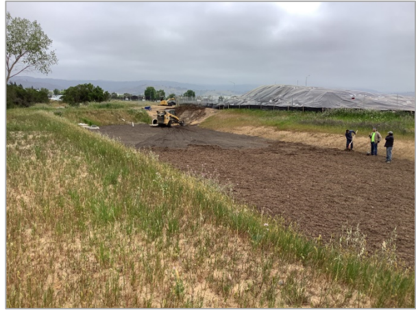
Photo 2. Construction of existing bioretention basin in southeast corner of site.
