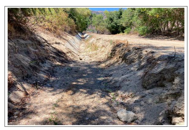
Photograph 7: June 2021. View of eroded earthen portion of Hill Street Channel looking upstream at concrete transition.
