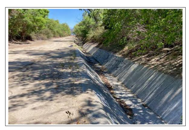
Photograph 6: June 2021. View depicting concrete portion of Hill Street Channel looking downstream towards Lake Elsinore. Note the transition to earthen channel in background.
