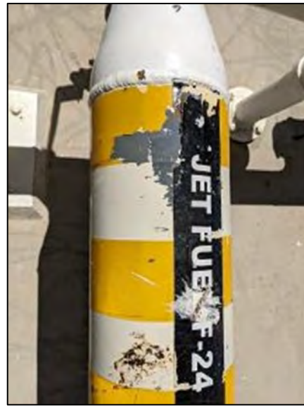
Photos 3 and 4 Raven Caused Corrosion of Facilities at SELF
