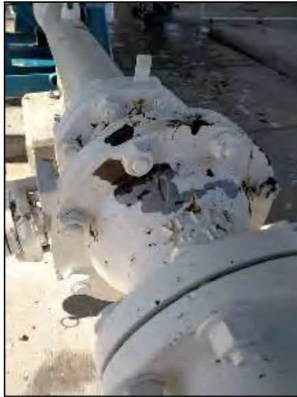
Photos 3 and 4 Raven Caused Corrosion of Facilities at SELF
