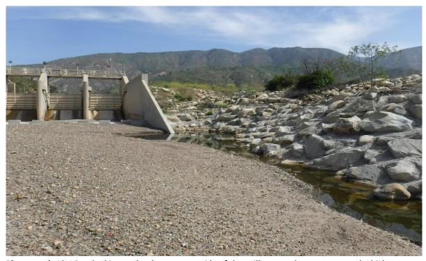
**Photograph 10.** View looking at the downstream side of the spillway, at the entrance pool which was completely filled in with sediment following storms post-Thomas Fire (May 2, 2019).
