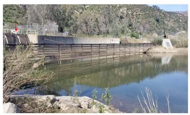
**Photograph 8.** View of the timber debris fence and high-flow fish exit (black arrow). The headworks is shown in back of the fence, denoted with a red arrow (February 4, 2020).
