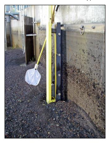
Photo 14- Sediment inundating fish screens and brushes in Robles Diversion screenbay
