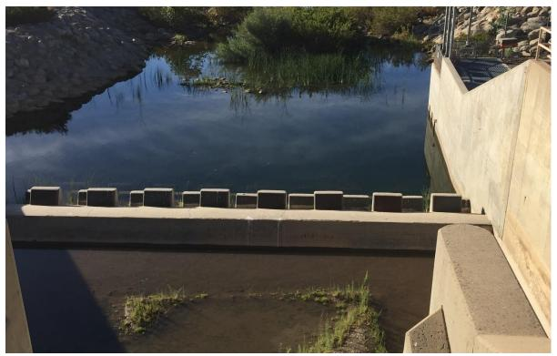
**Photograph 9.** View of the baffled apron downstream of the spillway, at the beginning of the entrance pool (December 13, 2019).
