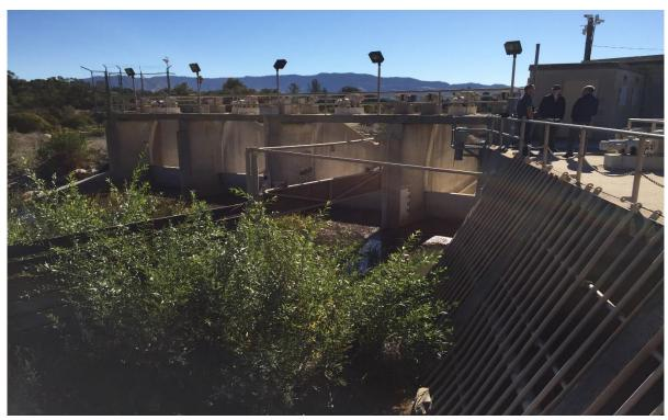
Photograph 7. View of upstream side of the spillway, radial gates and headworks (December 13, 2019).
