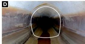
Tunneled, Cast-in-Place Pipe (Hoseshoe Shaped) 20-ft Sections; Cross-Sectional Area = 29.9 SF
