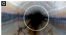
72-inch Concrete Pipe (Non-Cylinder) 16-ft Lay Lengths; Cross-Sectional Area = 28.3 SF
