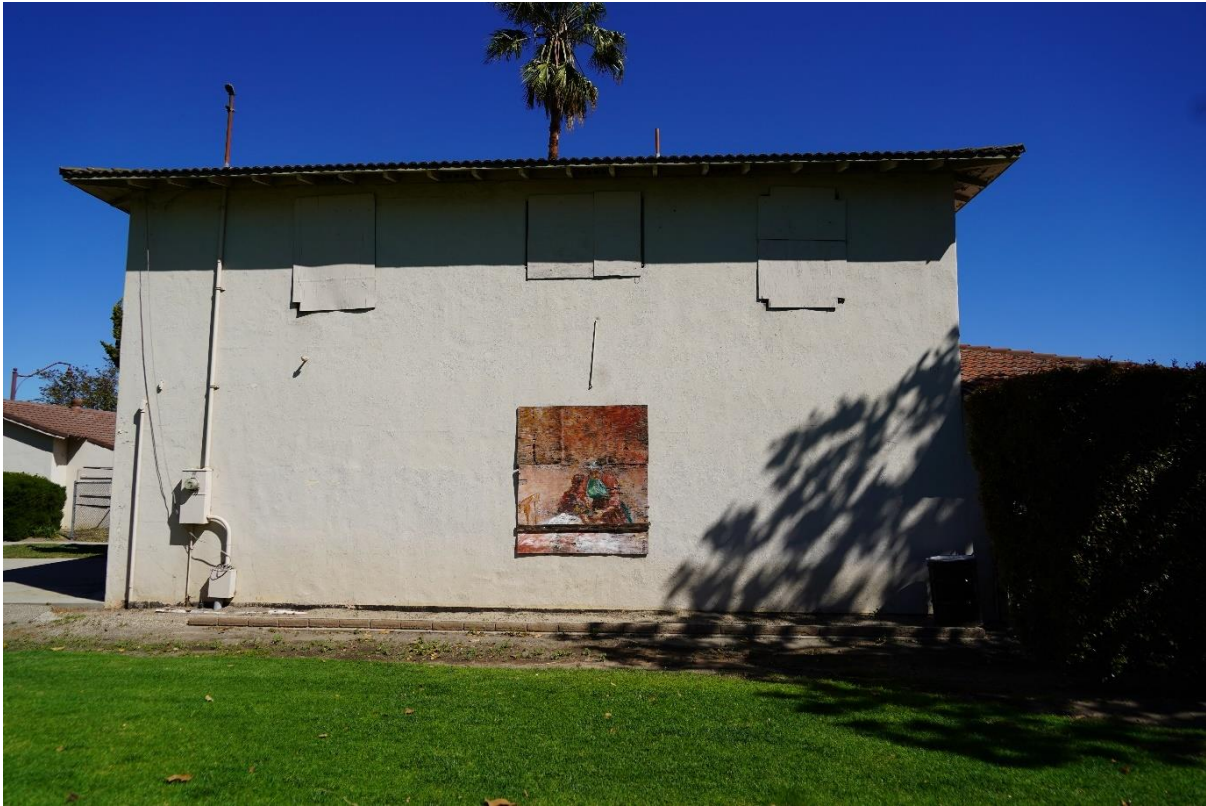
Figure 23 Boarded Window With Painting on West Elevation of Fire Station Garage
