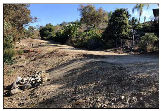
PHOTOGRAPH 3 Overview of Asphalt Water Crossing with Rip Rap, Looking East-Southeast
