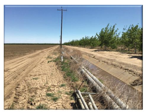
Plate 5. Looking east along irrigation canal on the southern border of the project. This concrete-lined canal is considered a permanent water conveyance feature. The area referred to as incidental to agriculture includes the canal, the dirt access road along the field border, and the ruderal area between the canal and the dirt road.
