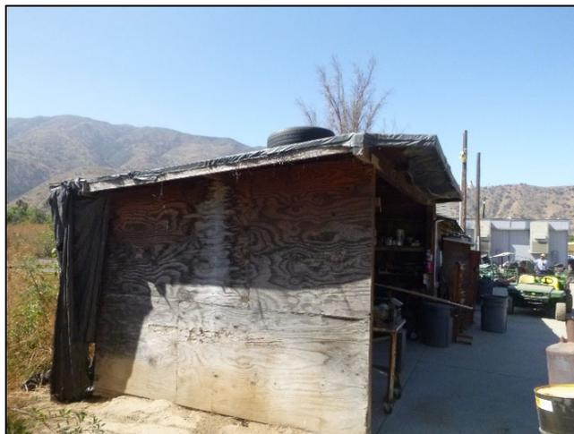
Figure 2      North elevation of Building 1, looking southwest. Note the more recent plywood siding and the new cement slab (Mills et al. 2019: Roll 3877-02-dm, Frame #14).
